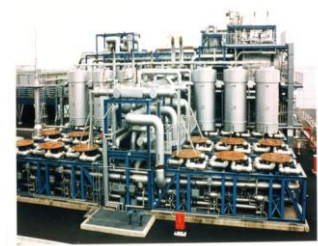
TEPCO 601 11MW FC POWER PLANT
